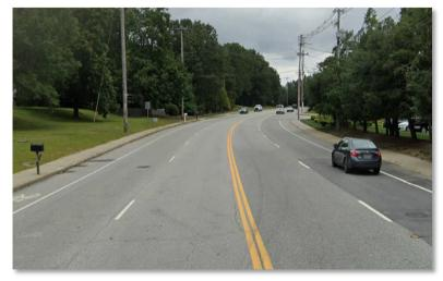
come to a stop prior to reaching an object in its travel path and avoid a collision. The available and required SSD are a function of the roadway geometry and design speed respectively, and are factored in when determining the appropriate and safe location of a site driveway or roadway intersection.
