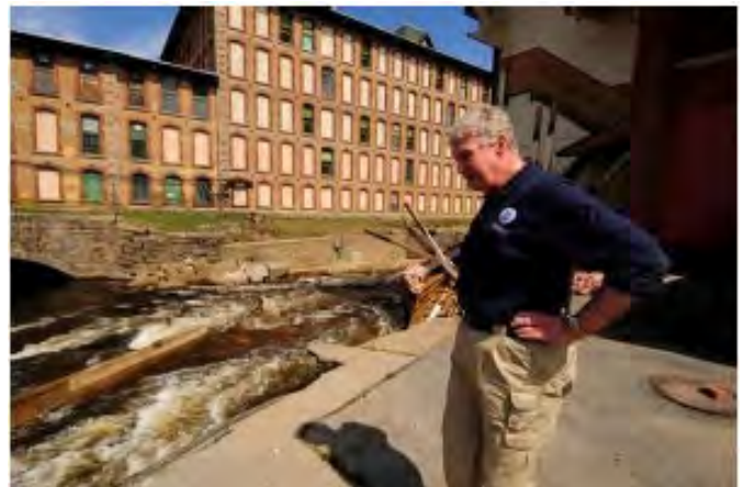
Figure 8- Historic Coventry mill building downstream of damaged bridge and dam- April 2010.
