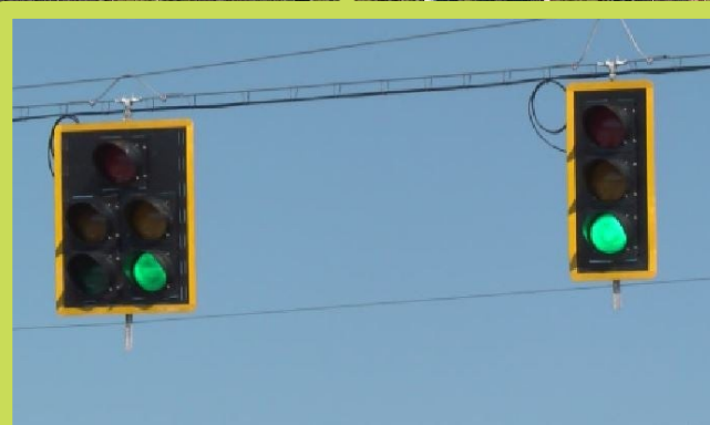
Example of traffic signals with backplates to increase luminance of lights
