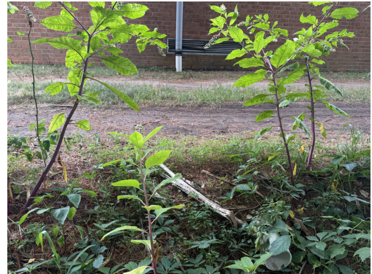
Existing condition downspout and outlet
