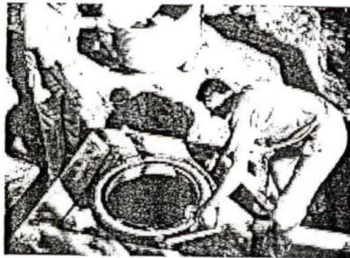
Your contractor should install access risers to grade on your septic tank.
