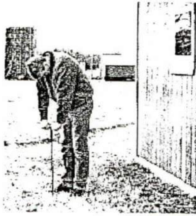
Locate the septic tank by probing with a metal rod. Be sure to avoid underground electric lines. Do not probe where there may be underground electric lines.
