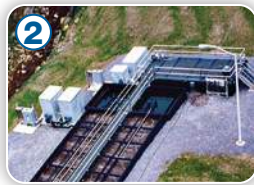
① Above-ground HRAS UniSystem® for industrial wastewater treatment at a food processing facility, ② In-Ground Air UniSystem® for municipal wastewater treatment with tertiary filters and UV disinfection, ③ Custom-engineered circular tank UniSystem® with internal clarifier for treating 190,000 gpd of wastewater
