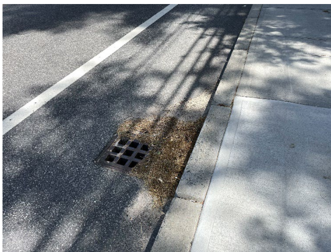
Catch basin observed along Arnold Road
