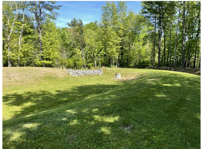
Sandy Bottom Road Infiltration Basin
