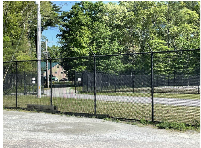
Figure 1 - View of the Mishnock Treatment Facility
