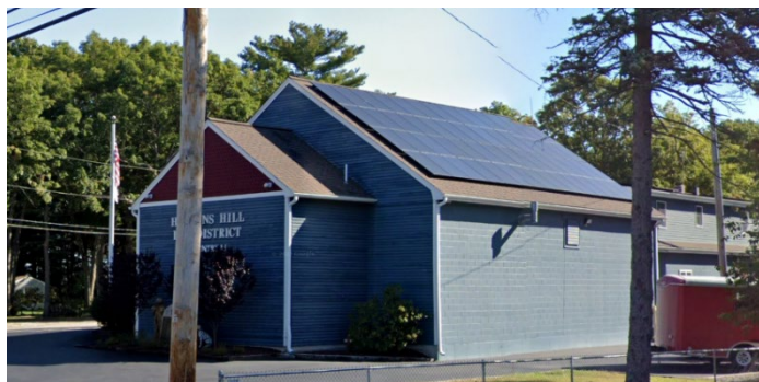
Figure 8.1 - Hopkins Hill Fire District Roof-Mounted Solar Array, Google Maps Streetview, 2019
