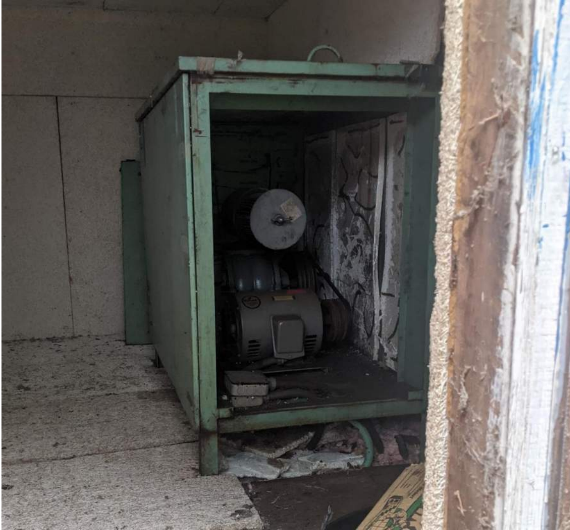
Figure 4: OWTS Compressor
