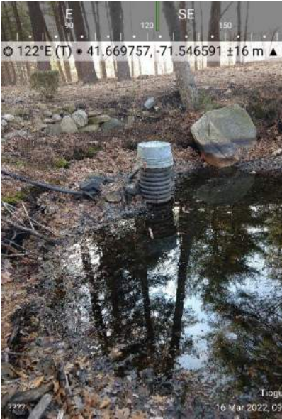
Figure 8a: A suspected water intake located south of Tiffany Rd
