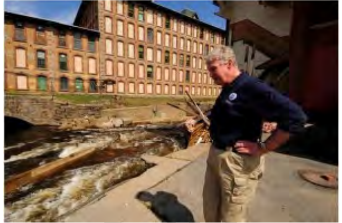
Figure 8- Historic Coventry mill building downstream of damaged bridge and dam- April 2010.
