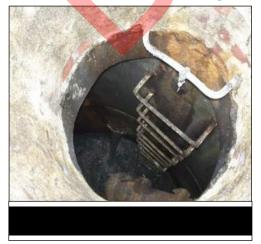
prior to pump operation, allowing for proper pumping and level control, maintaining sufficient submergence of the pump suction inlet, preventing excessive deposition of solids, and providing ventilation of incoming sewer gases. Dependent upon the size and use of the facility, the installation of pump protection (shredder) in the wet well is generally recommended to protect pumps from clogging.
