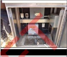
The electrical control system components are in good condition. There was a totalized flow of 240,175,520 gallons but no flow during our observation. There was no flow totalizer at the Woodland Pump Station to compare values.
