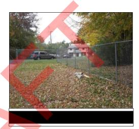
In general, the ground slopes towards the rear of the site (from north to south); however, there are minor soil settlements throughout the site. Much of the soil along the west side of the building is level or slopes towards the building. This does not allow for provide positive drainage away from the building. This condition can allow rainwater to accumulate against the foundation and may allow water to migrate through the foundation wall into the building.
