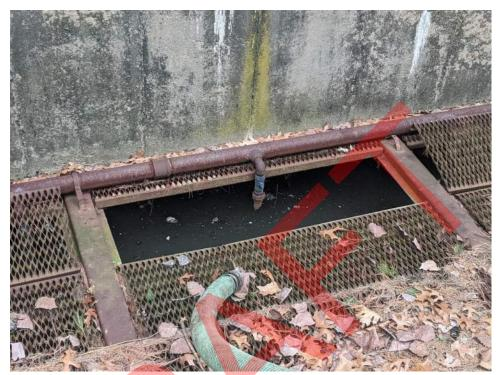
Figure 2: Deteriorated Aeration Piping
