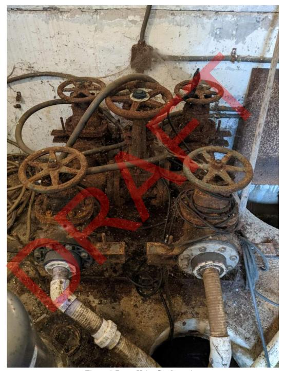
Figure 6: Pump Valve Configuration
