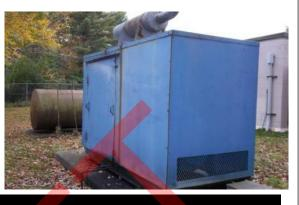
The fuel tank for the generator is located next to the generator. The tank is a single wall steel tank (approximately 1,000 gallons) on a concrete pad (5 foot x 12 foot).
