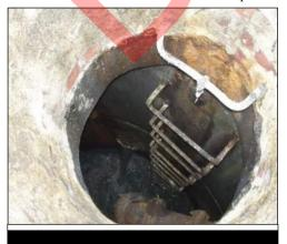
prior to pump operation, allowing for proper pumping and level control, maintaining sufficient submergence of the pump suction inlet, preventing excessive deposition of solids, and providing ventilation of incoming sewer gases. Dependent upon the size and use of the facility, the installation of pump protection (shredder) in the wet well is generally recommended to protect pumps from clogging.
