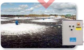
Aqua-Jet<sup>®</sup> aerator and typical Definite Purpose Control Panel.
