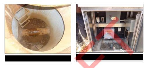
The electrical control system components are in good condition. There was a totalized flow of 240,175,520 gallons but no flow during our observation. There was no flow totalizer at the Woodland Pump Station to compare values.
