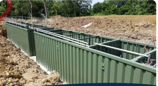
Multi-train factory-built ADDIGEST® installations are available, as seen in this picture.
