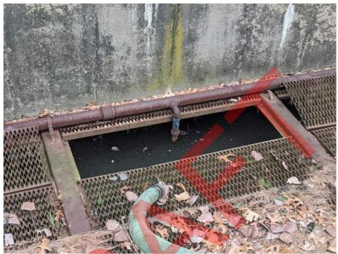
Figure 2: Deteriorated Aeration Piping
