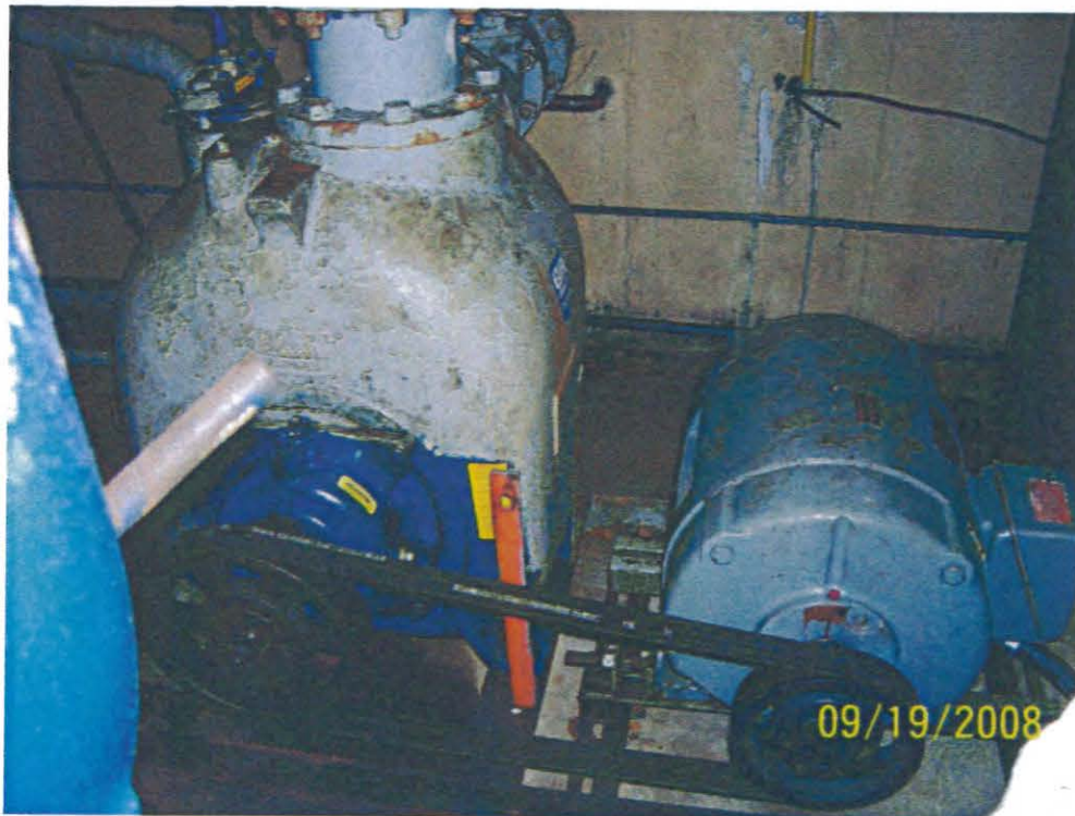
Figure 6: Pump in process of being repaired (since completed)
